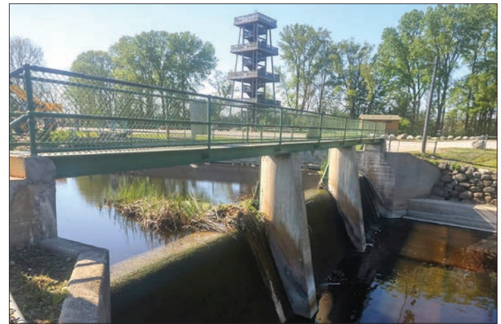
THE OLD DAM , showing a cattail mat hung up at the edge. The new dam is designed to allow for improved cattail control. - Photo by Friends of the Broughton Sheboygan Marsh
