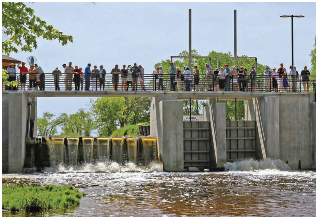
THE SHEBOYGAN MARSH'S NEW DAM was toured by guests to a dedication ceremony Sunday May 19. The state-of-the art structure allows for improved ecosystem management - with cattail mat control one major driver of the project. -Beacon photo by Sarah Hall
