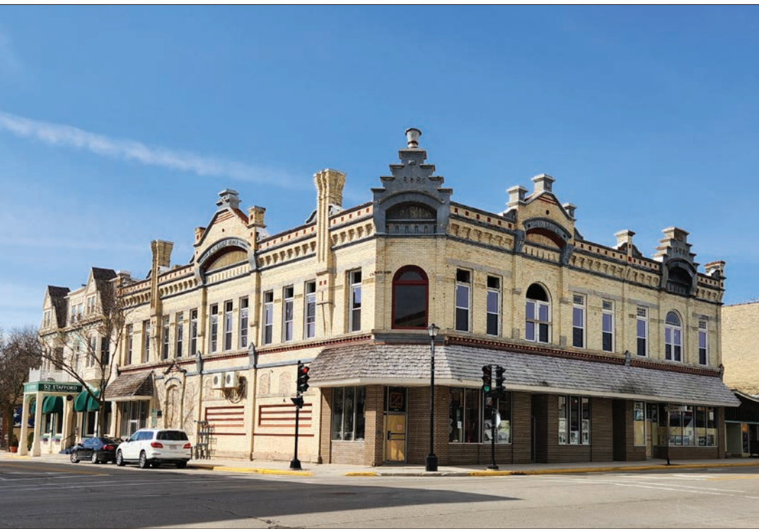
THE H.C. LAACK BUILDING at the southwest corner of Mill and Stafford Streets is set to be purchased and restored by the Gentine family of Plymouth. The purchase also includes the Laack Hotel, currently 52 Stafford, which is on the left in the photo. –Beacon photo by Kay Preissner
