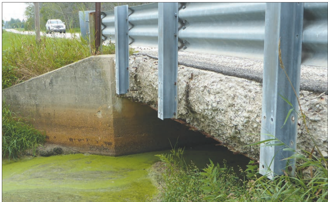
THE CRUMBLING EDGES and loose railing struts are clearly visible on bridge east of Hingham on County Road W slated for repair. Neighboring property owners say it traps runoff which floods cropland. — Beacon photo by Ian Johanson
